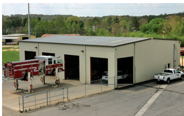
Motor Maintenance Facility
